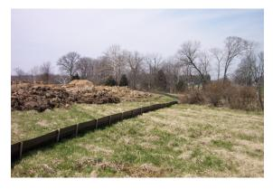
Drain Filtering / Sediment trap
